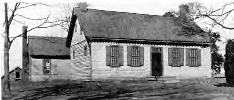
Slate Hill, the plantation house of Nathaniel Venable. At left is the plantation office, in which the Presbytery met to found the College. It now stands on campus.
